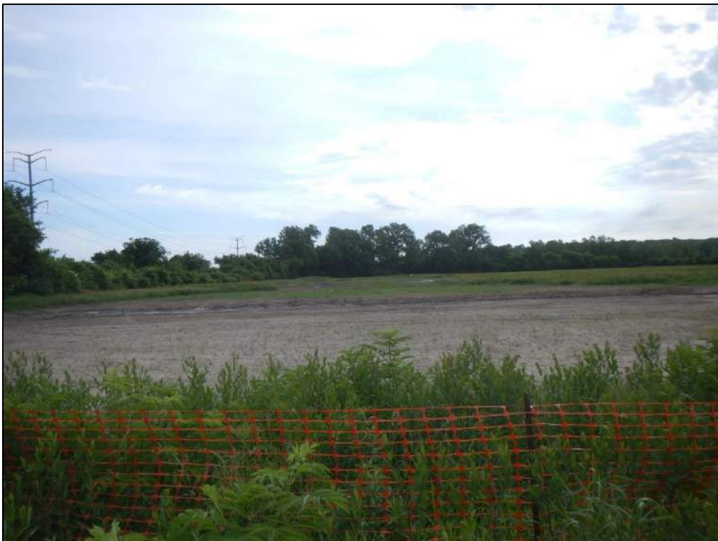
Photograph 12. Overview of disturbed area, graded area. View to the northeast.
