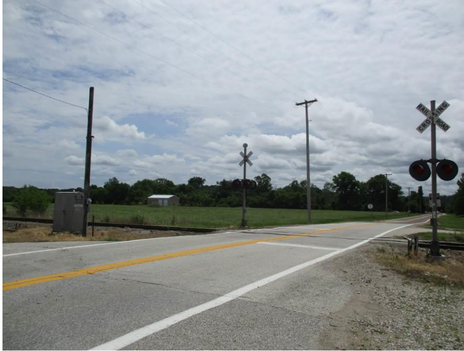
Photo 4. View to the southeast from Marine Avenue toward railroad crossing, the project site and the maintenance shed
